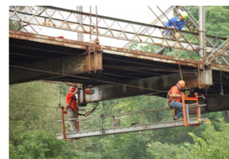
Fig. 3 Structure based access on tensioned cables. Not limited to bridges, rigging is available to inspect piers, towers, dams and tall buildings.
