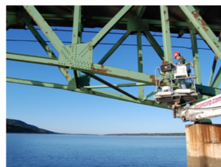
Fig. 2 Boats with working heights up to 88ft with shallow water capabilities of less than a foot
